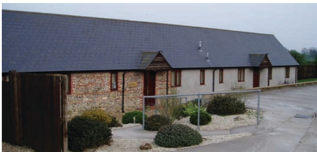
Units at Manor Farm
